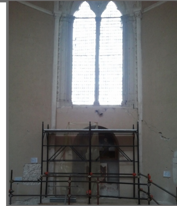
Internal view of the apse
